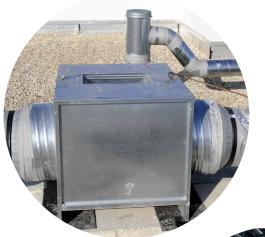
When positioned on a ventilation box, the Delta P lets one monitor, at a distance, the proper operation of the system, and it will be alerted in the event of a malfunction (electrical, breakdown, fouling...).
