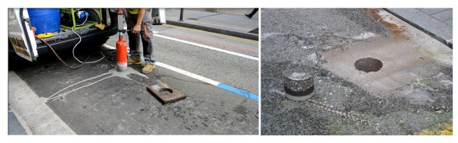
Figure : Making a hole in the pavement
