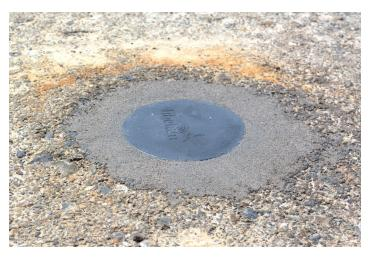
Figure : Final Epoxy application
