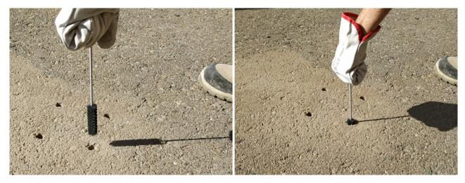
*Figure : Brush the hole (step 3)*
