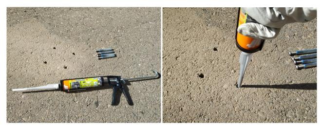
Figure : Inject chemical fixing adhesive (step 5)
