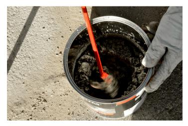
Figure : Preparing the Epoxy resin mixture
