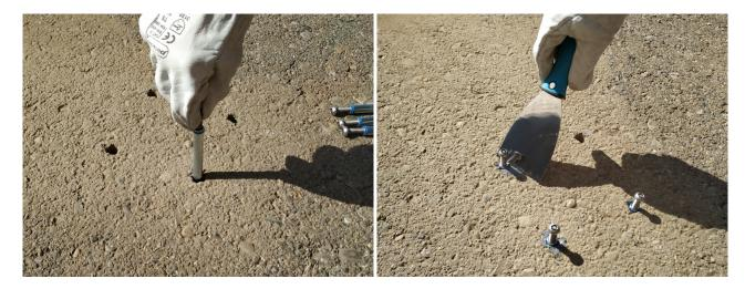
*Figure : Insert the anchors (step 6)*
