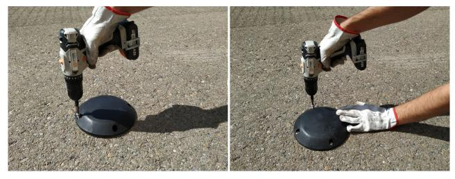
Figure : Screw the node
