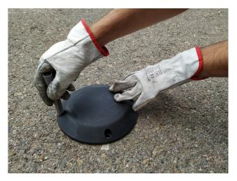
Figure : Marking the holes for the node
